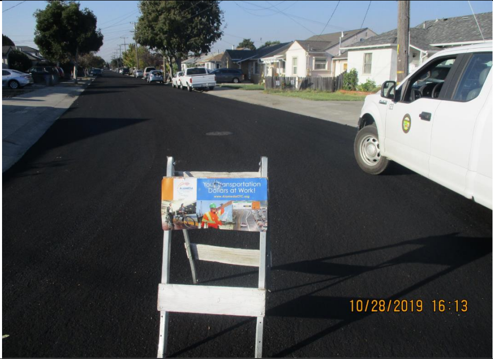
COMPLETED SLURRY SEAL ON PIERCE AVENUE
