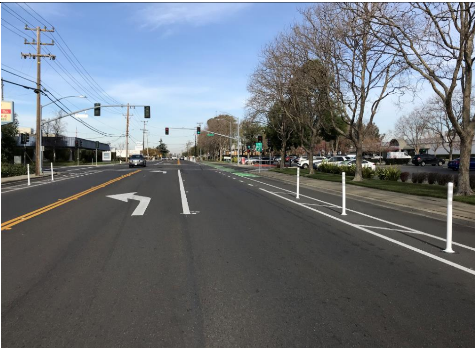
COMPLETED CAPE SEAL WITH NEW CLASS IV BIKE LANES ON ALVARADO STREET
